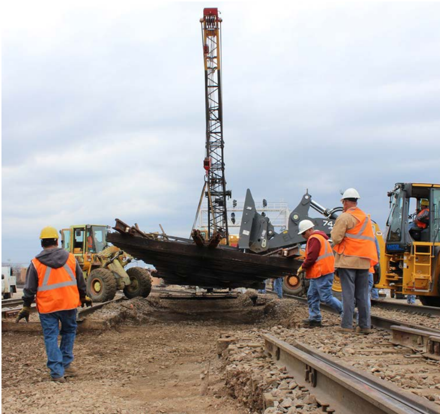
Track work at A-5 Junction in Chicago
