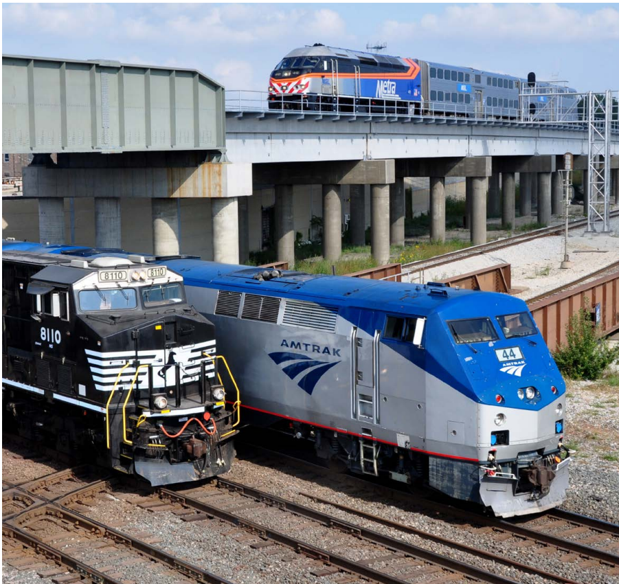
Construction of the Englewood Flyover has eliminated conflicts between RI trains and freight and Amtrak trains at a critical rail junction near 63rd Street in Chicago
